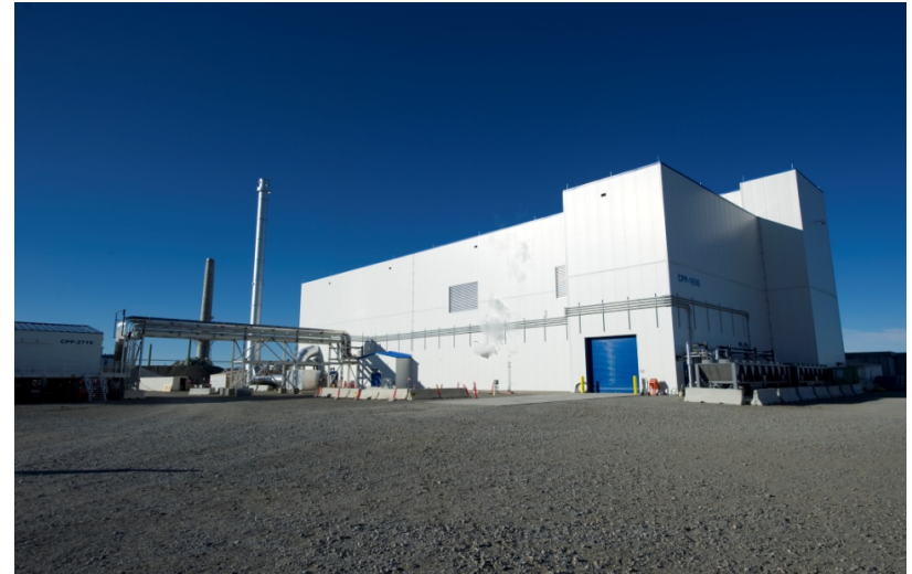
Integrated Waste Treatment Unit
